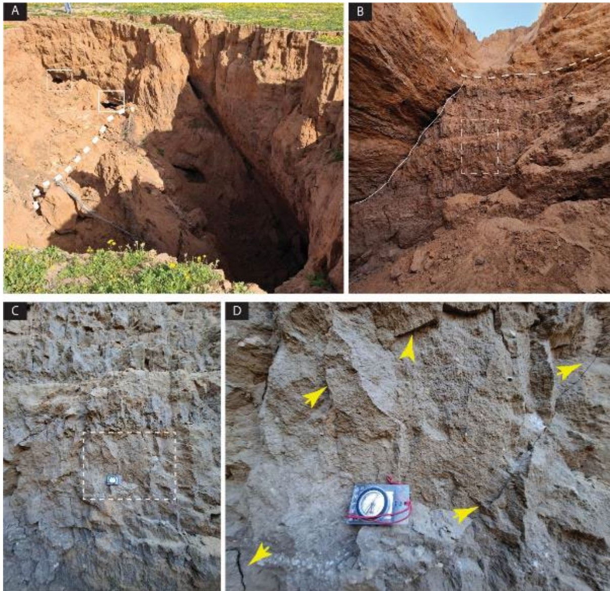
Figure 5. Visible characteristics of the exposed soil section: A) the trench made by the collapsed soil, it shows the position of the caliche (marked by the dashed line) and the erosion cavity below the caliche (the rectangles); B) representative view of the soil section, the dashed line separates the upper soil from the subsoil, the inclined line traces a large fracture in subsoil, the dashed rectangle is a view in the subsoil magnified in C) which shows the heterogeneity within the subsoil, represented by the presences of sandy patches/layers within the clay-dominated grey soil; D) close view from ( the rectangle in C) shows that the subsoil is intensely fractures, the arrows points to open fractures and fracture faces
