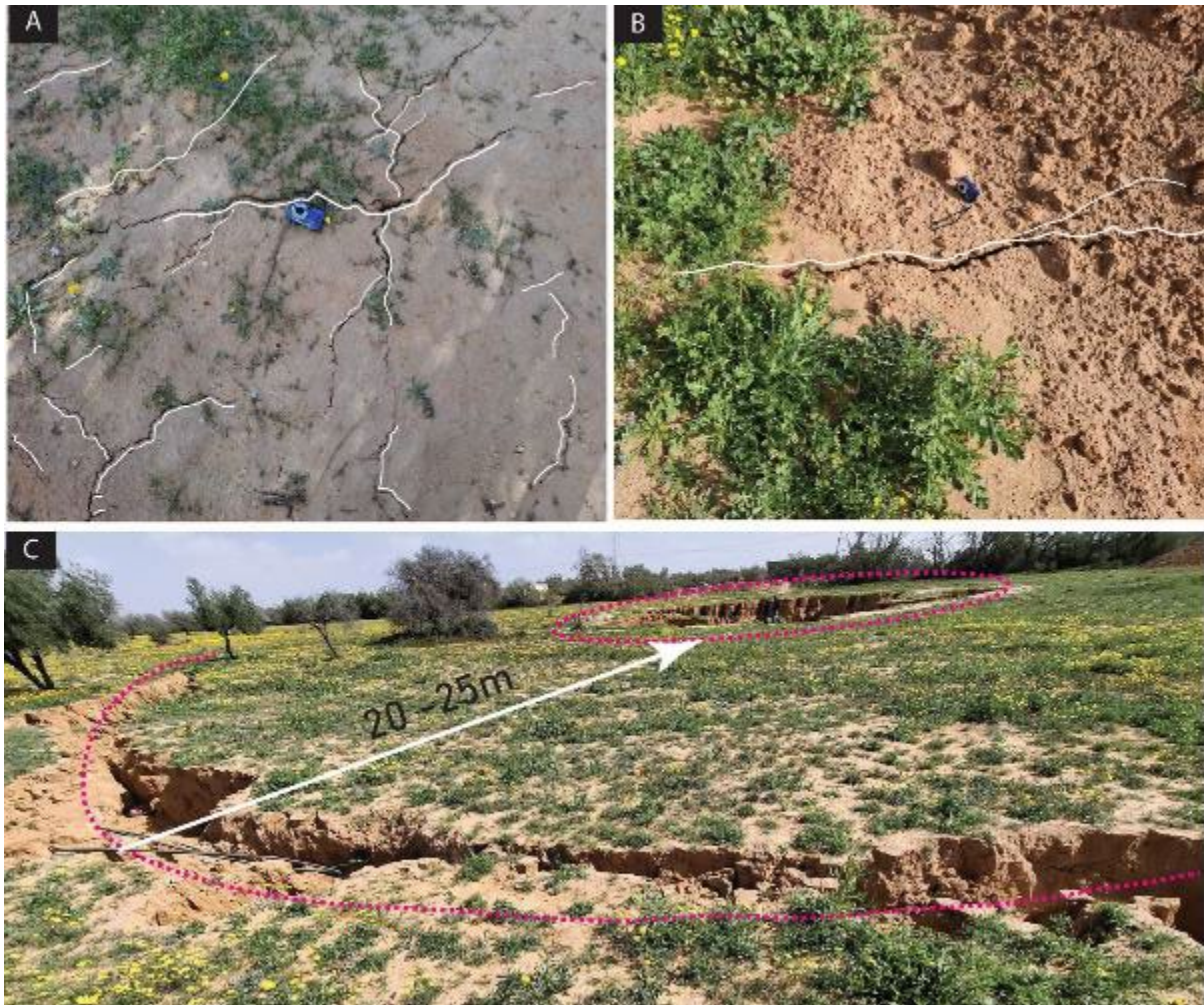
Figure 3. The cracks morphology and size: A) the commonest pattern taken by the small cracks (usually at a distance from large cracks (camera for scale); B) elongated cracks usually attached to larger crack; C) large; several tens of meters semicircular cracks (dashed line) centered around the deepest collapse. Subtle inclination of the ground can be noted from the crack toward the collapsed spot (dashed circle).
