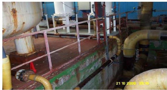
Figure 3. Coagulation-flocculation tanks [6]
