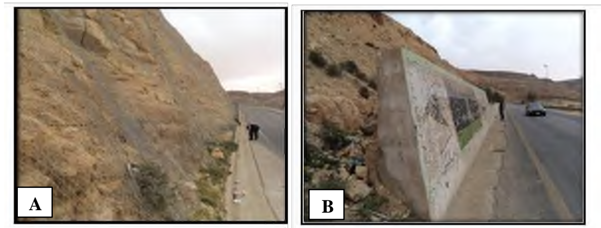
Photograph 3 (A - B). Showing the use of metal nets fences and concrete walls to prevent the rockfalls of Ain Tobi Member.
